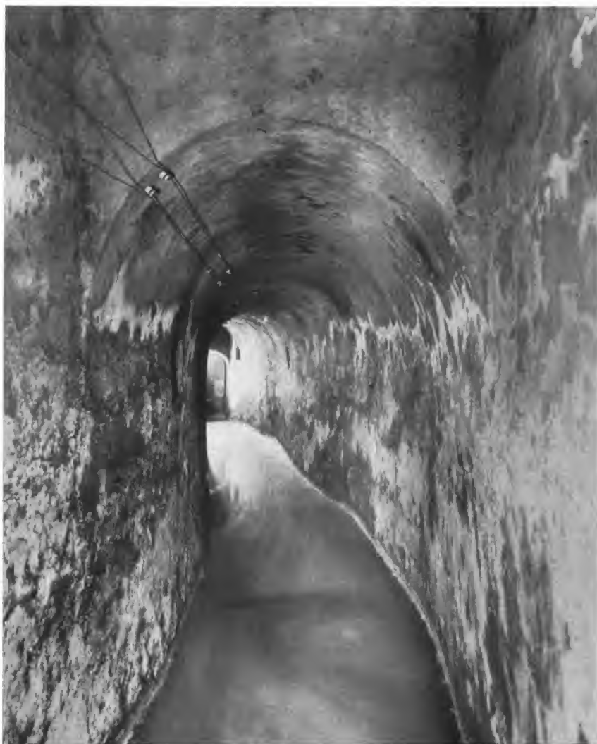
Fig. 130 — S. Lorenzo in Fonte. Corridor leading to well-house (Photo: Sansaini)
